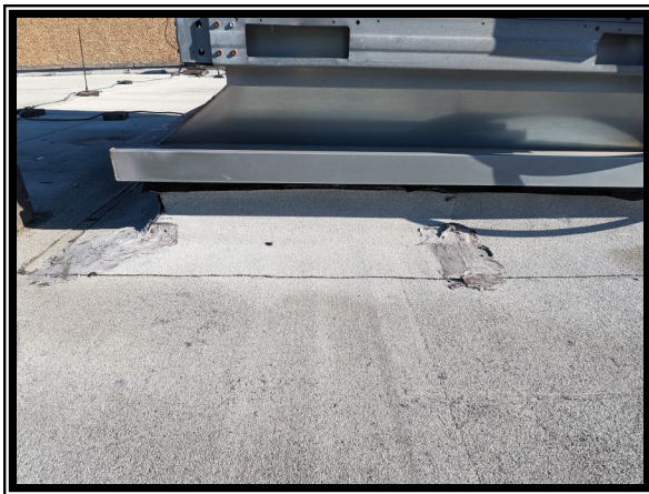
Photo #3 View Depicting Curb Sealants of Roof Section A
