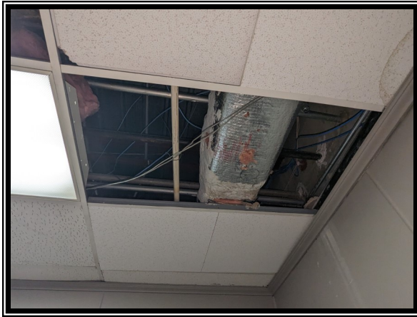
Photo #9 No Asbestos Detected in Ceiling Tiles or HVAC Duct Materials in the Office Areas
