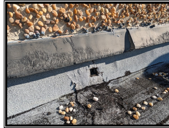
Photo #2 No Asbestos Detected in Base Layers or Metal Flashing Materials of Roof Section A
