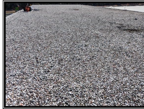
Photo #6 No Asbestos Detected in Built-up Roofing Layers of Roof Section D
