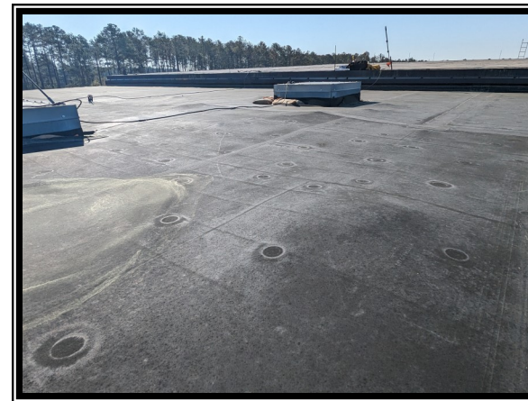
Photo #4 No Asbestos Detected in EPDM Roof System of Roof Section C.
