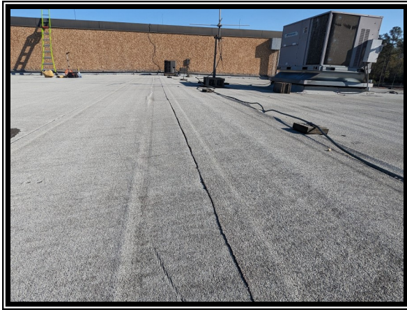
Photo #1 No Asbestos Detected in Roofing Layers of Roof Section A
