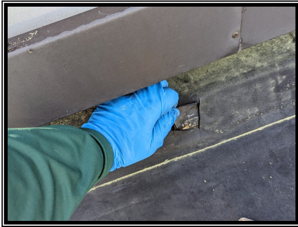
Photo #5 No Asbestos Detected in Wall/Curb Base Sealant Layers of Roof Section C
