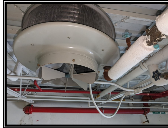
Photo #10 No Asbestos Detected in Ceiling-mounted Fan Coils' Pipe Wrap Material
